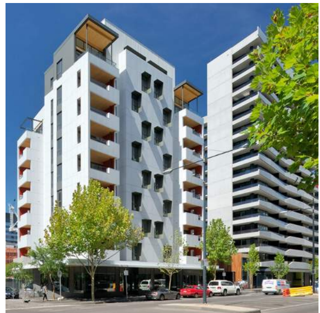
Forte building – Docklands, Melbourne. 10-storey apartment block made from cross-laminated timber.
