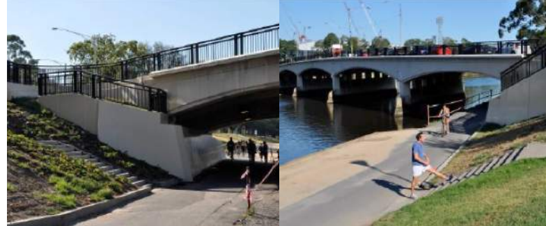
Retaining walls made from Zeobond's E-Crete at Swan St Bridge, Melbourne.
