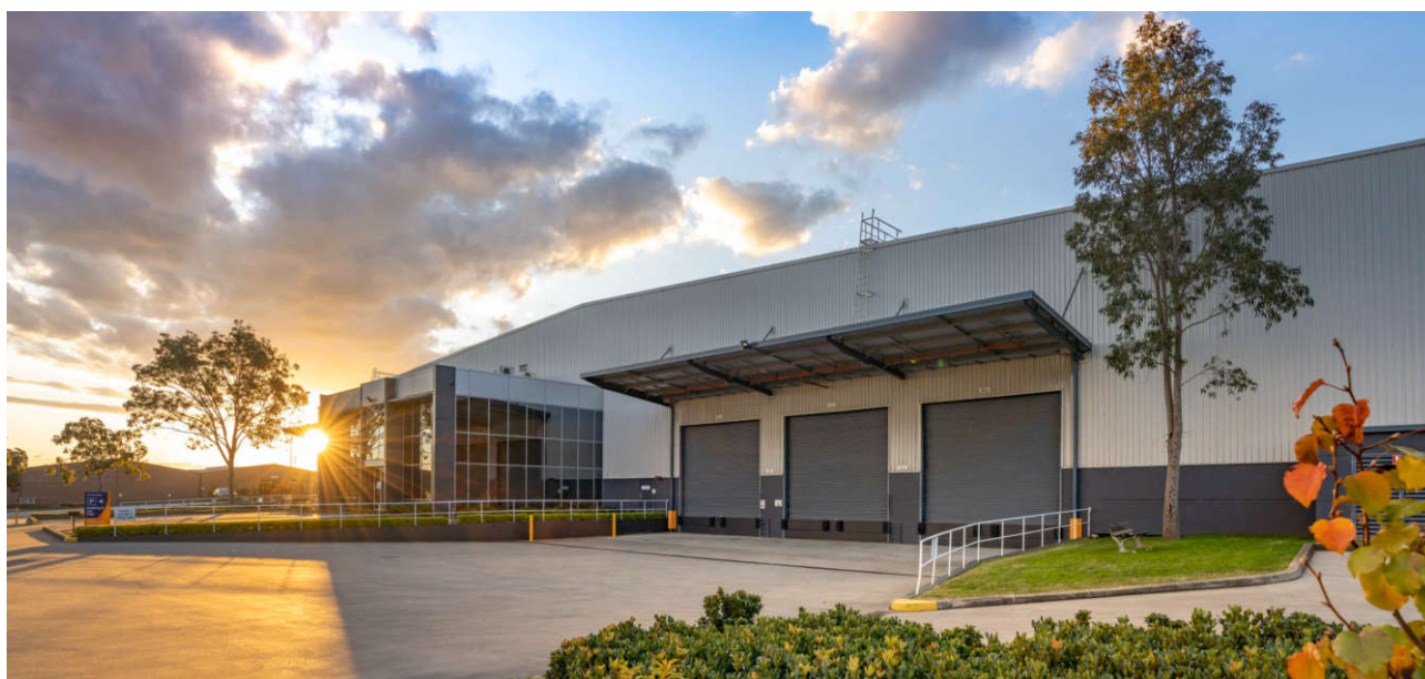
Yennora Distribution Centre, NSW
