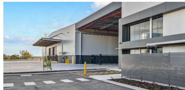
18 Gorrick Court, Bundamba, QLD Completed May 2022 Fair Value 1 $42.5m | GQLT (GPT 50.1%)
