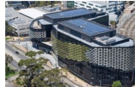
Building 3, 570 Swan Street, Richmond, Victoria
