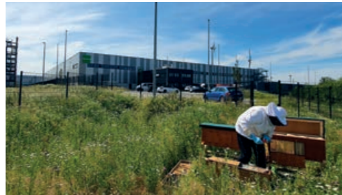
Mönchengladbach IV Logistics Centre, Mönchengladbach, Germany.
