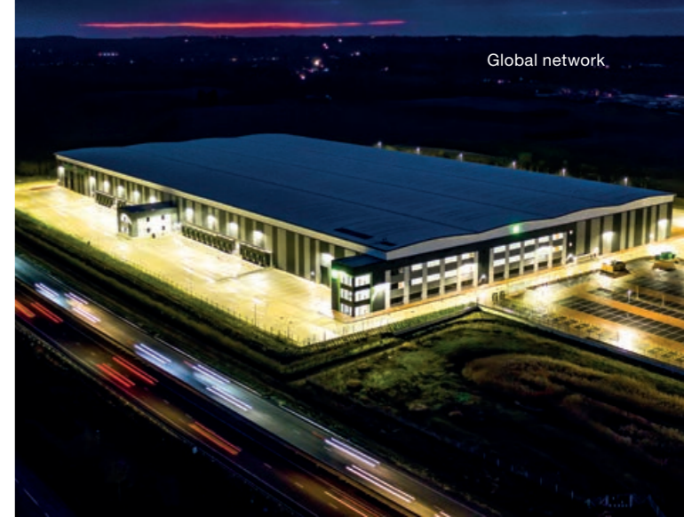
Bedford Commercial Park, Bedford, United Kingdom.
