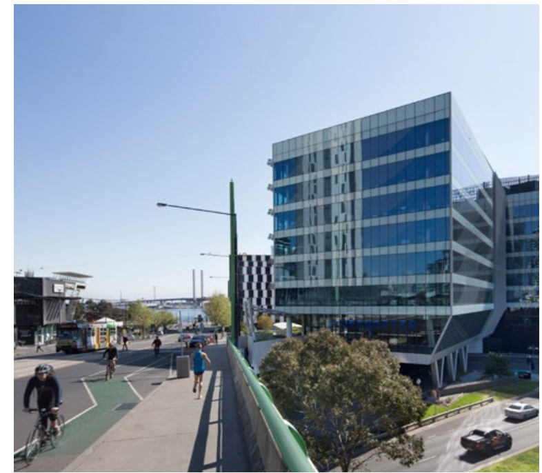
990 La Trobe Street, Docklands, Melbourne Vic 6.0 Star NABERS Energy 6.0 Star NABERS Water
