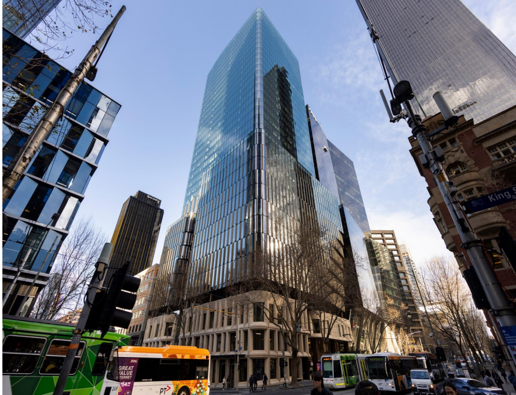
555 Collins Street, Melbourne (CPOF)
