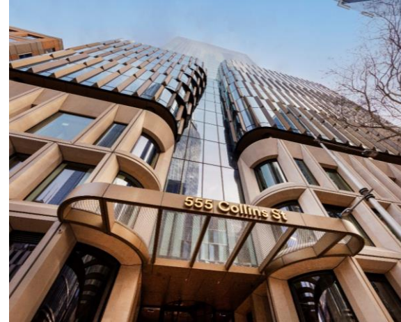
555 Collins Street, Melbourne (CPOF)
