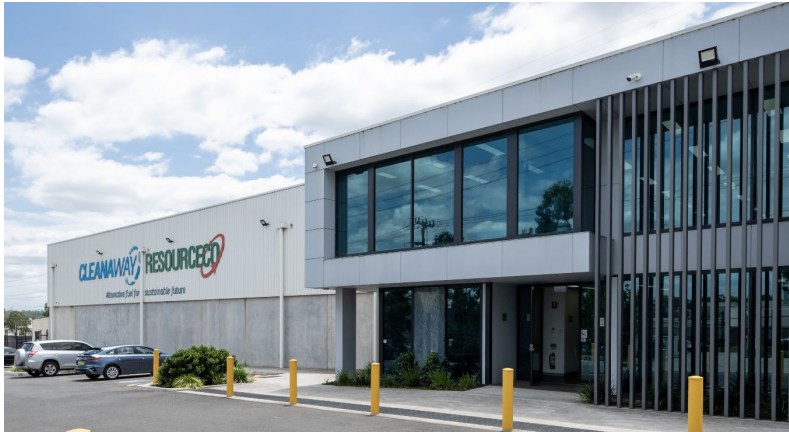
Cleanaway & ResourceCo Facility, Sydney NSW
