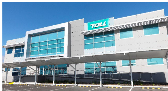
Toll Altona North, VIC
