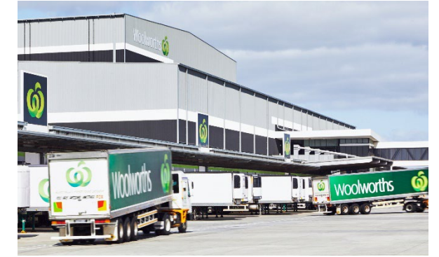
Woolworths Distribution Centre, Dandenong, Melbourne
