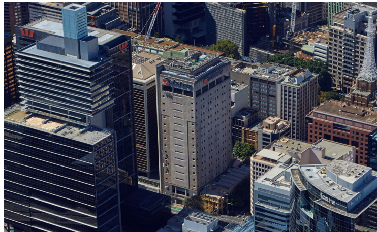
Kent Street Exchange, NSW
