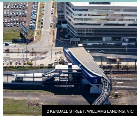
2 KENDALL STREET, WILLIAMS LANDING, VIC
