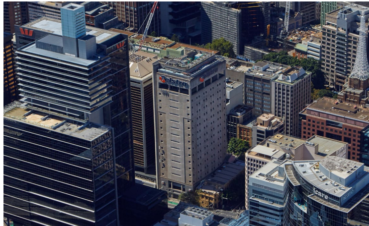
Kent Street Exchange, NSW
