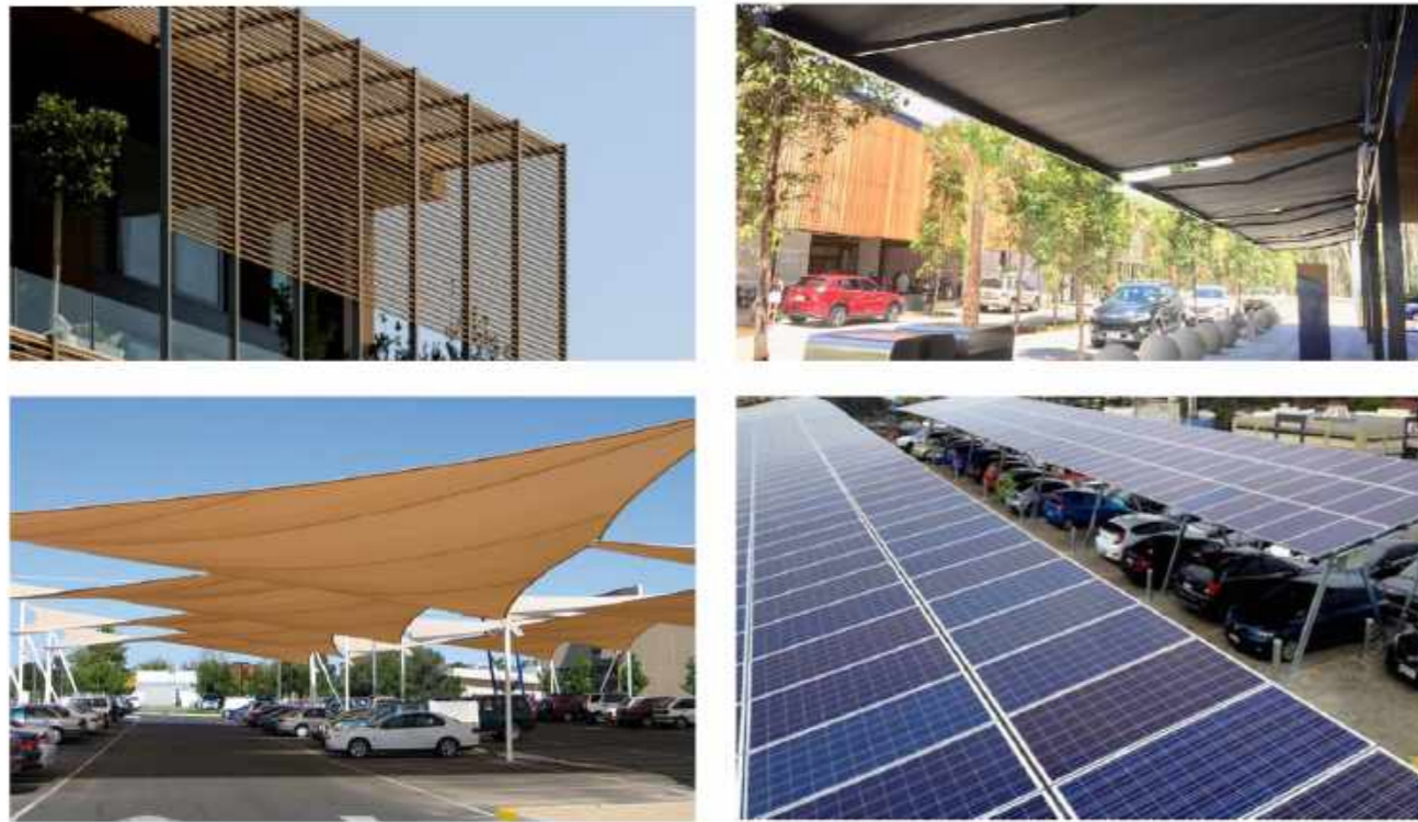
Figure 20. Examples of permanent and non-permanent shading structures (CRC for Low Carbon Living, 2017) – note the solar photovoltaic panels.
